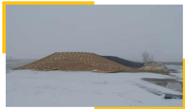
that imposed by the actual 55 mph wind. Therefore, while wind forces were a clear trigger of the failure given the structure's displacement to the east, it was reasonable to initially infer that an underlying issue in the structure's capacity to resist wind forces contributed to the failure.
